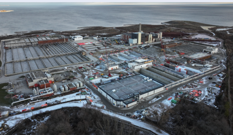
▲ Phase 2 construction in late 2025
