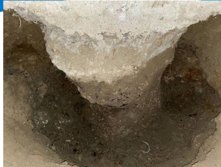
A close-up photograph of a concrete pile foundation. The pile is cylindrical and shows signs of weathering and discoloration. It is surrounded by a trench filled with dark, moist soil. At the base of the pile, there is a dark, reflective area that appears to be water or a void, possibly indicating a leak or a void in the foundation. The surrounding soil is uneven and appears to be a mix of dirt and small stones.
