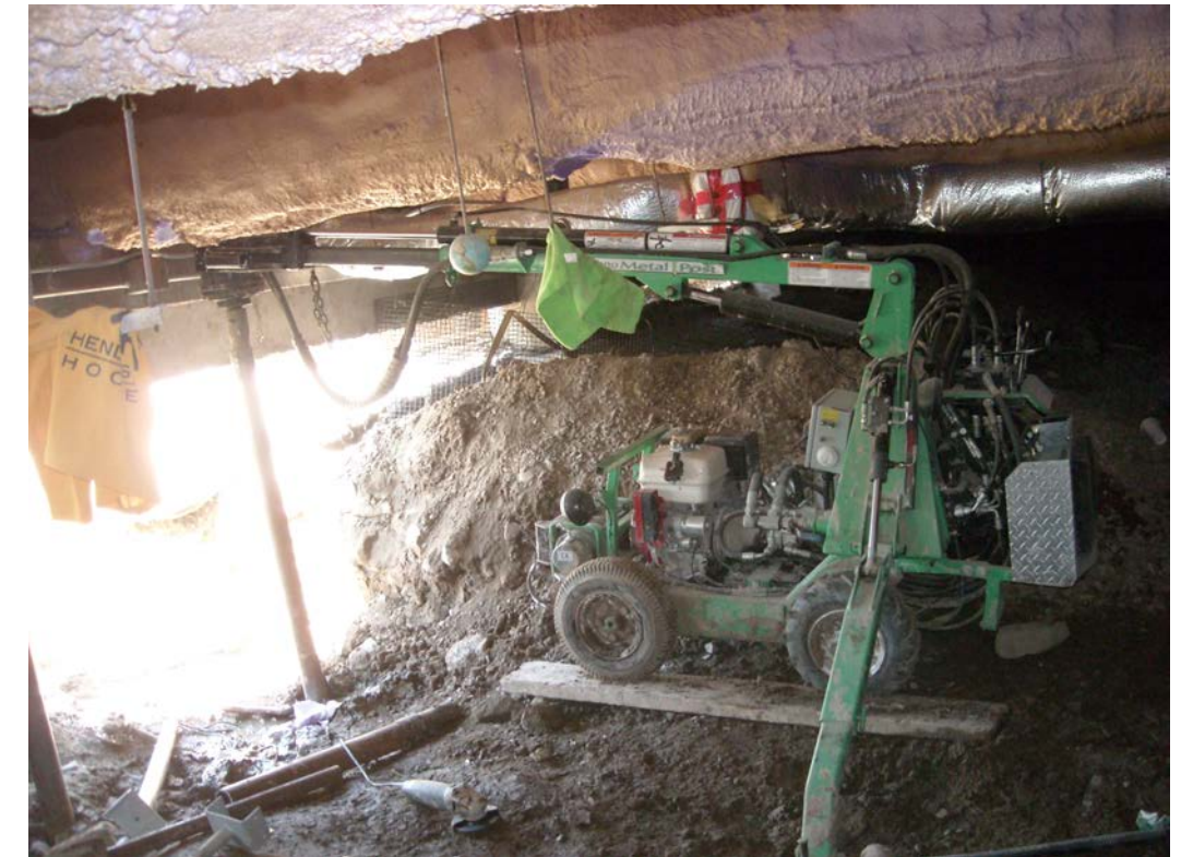
Installation of piles – exterior and under building crawl space
