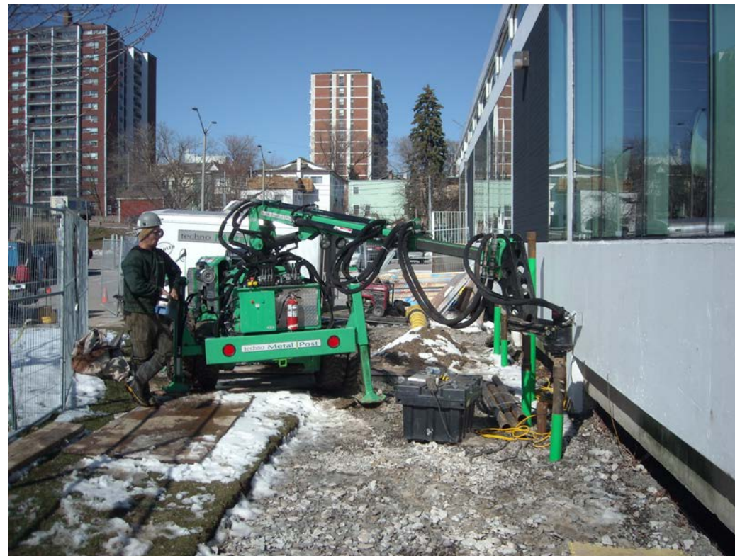
Installation of piles – exterior and under building crawl space
